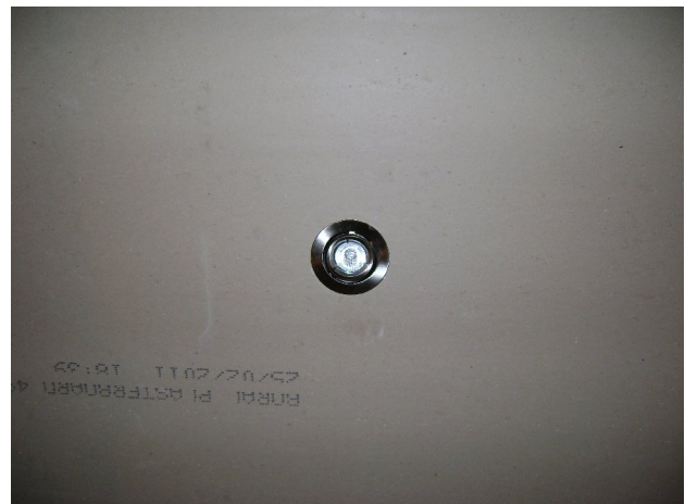
Figure 2.2: Downlight installation in plasterboard (from receiving chamber)
